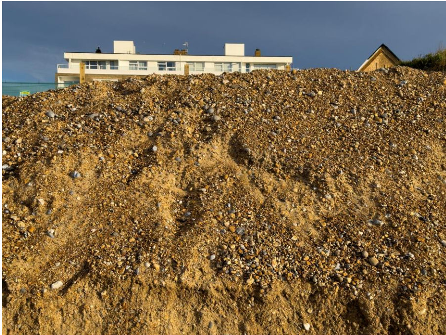
The Environment Agency’s giant stack of shingle at Cooden Beach Hotel is for use along the coast to prevent sea flooding.
